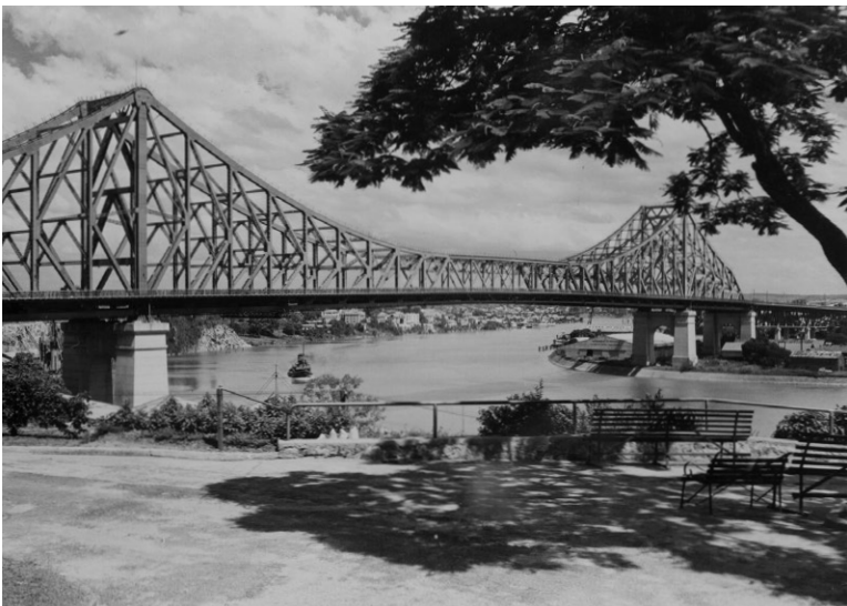
Story Bridge from Ivory Street, Brisbane City - 1949
